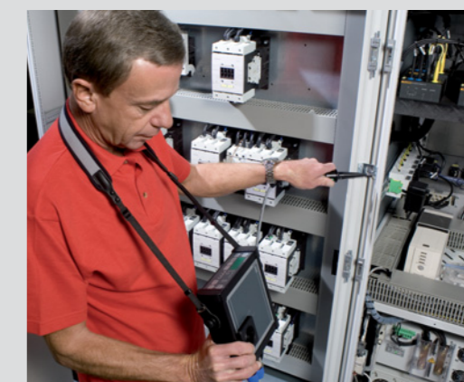
EN60204 test at a service cabinet
