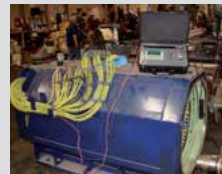
MTC2 light on a wind-power generator
